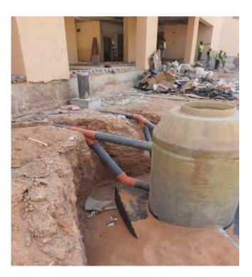
> HDPE Pipe Installation for portable & Irrigation water line.
