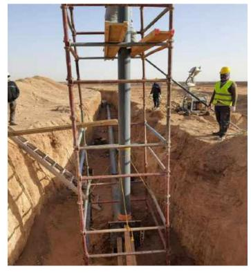
> GRP Manhole Installation with piping connection for Sewage.
