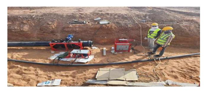
> HDPE **SADDLE TEE** Electro Fusion Joint Process for portable water line.
